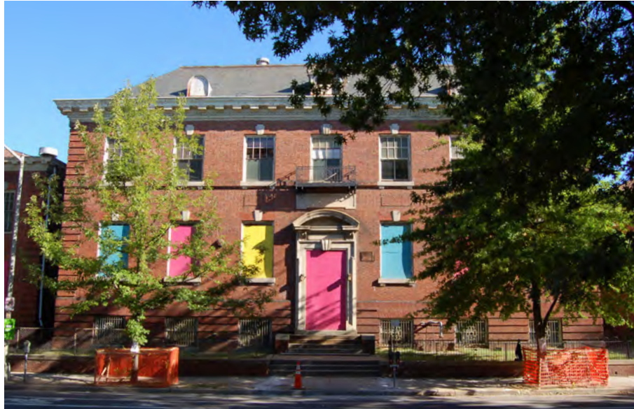
CENTRAL BUILDING - SOUTH ELEVATION (EXISTING CONDITIONS)
